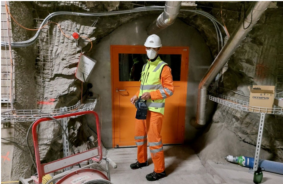
Figure 1: CD-A: C. Ostertag-Henning installing the new gas port next to the door of the Niche Closed Twin (Photo: G. Ziefle, BGR).
