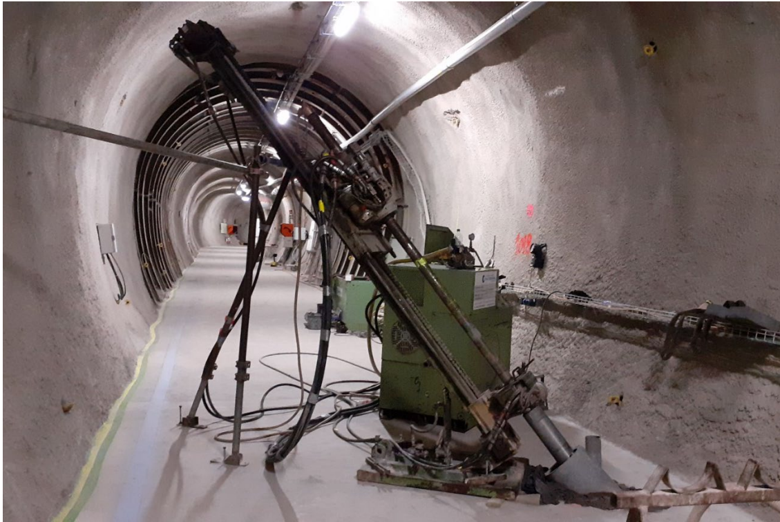
Figure 1: DR-D: Installation for BDR-D1 is ready (Photo: V. Regard, swisstopo).
