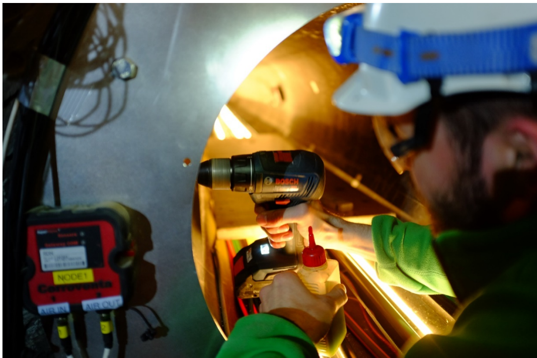
Figure 2: PF: A. Degiacomi drills the first few holes for the fibre-optic attachments inside the casing of BPF-7 (Photo: T. Steffen, swisstopo).
