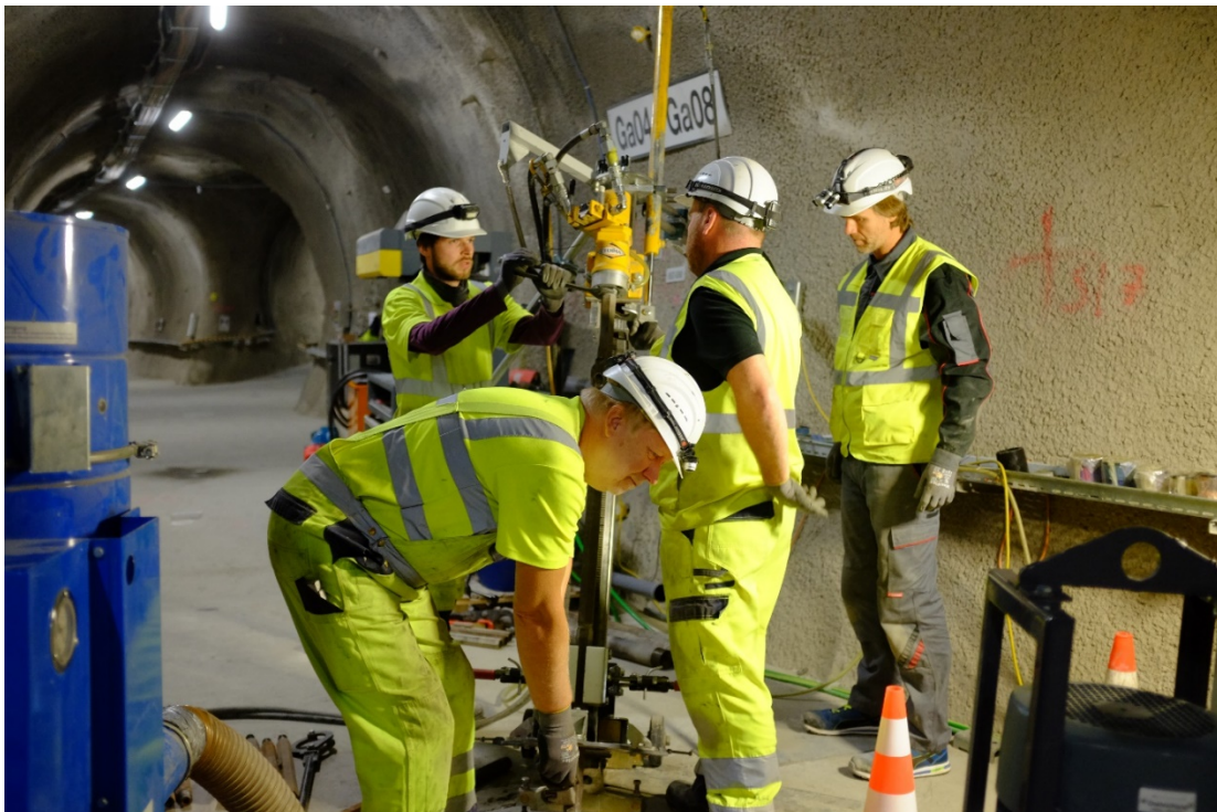
Figure 2: SW-A: The GRS-team retracting a core (Photo: S. Schefer, swisstopo).
