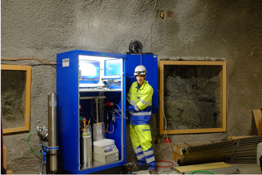
Figure 1: GT: Installation of the new cabinet (Photo: S. Schefer, swisstopo).
