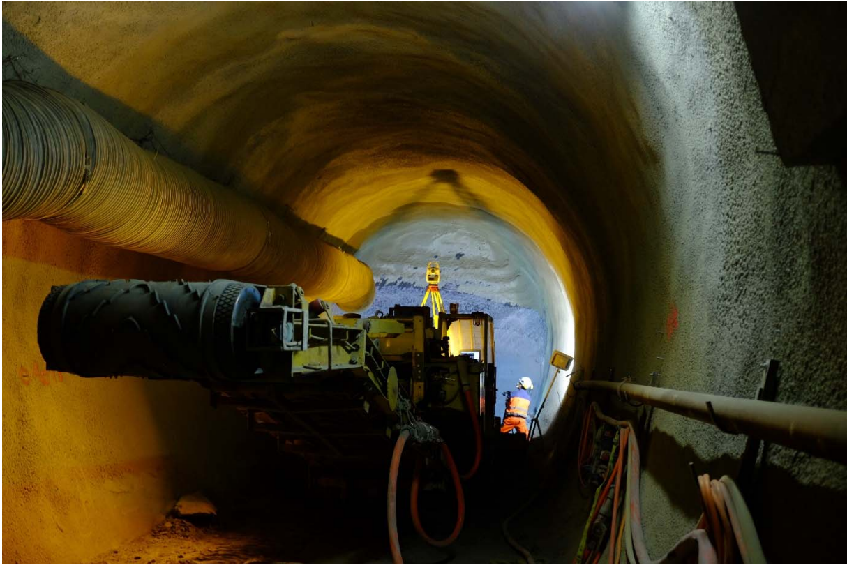
Figure 1: Ga18: D. Jaeggi (swisstopo) working his way around the roadheader to create a model of the tunnelfront. On top of the roadheader the theodolite, which is used to set up the coordinates of the model, can be observed (Photo: S. Schefer, swisstopo).
