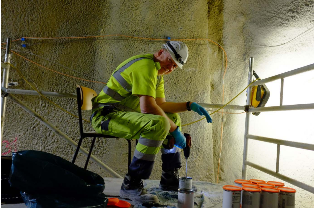
Figure 1: MB-A: M. Komischke (GRS) preparing resin for the sealing of BMB-A24 (Photo: R. Raselli, swisstopo).
