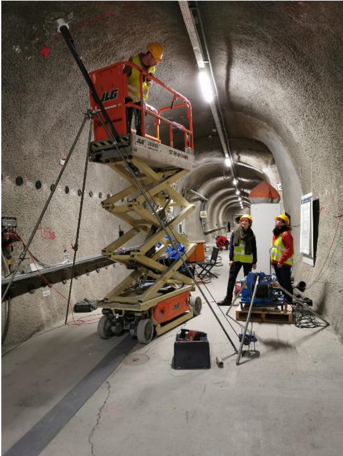
Figure 1: SE-P: The ETH-team logging an ascending borehole (Photo: S. Lüchinger, ETH)
