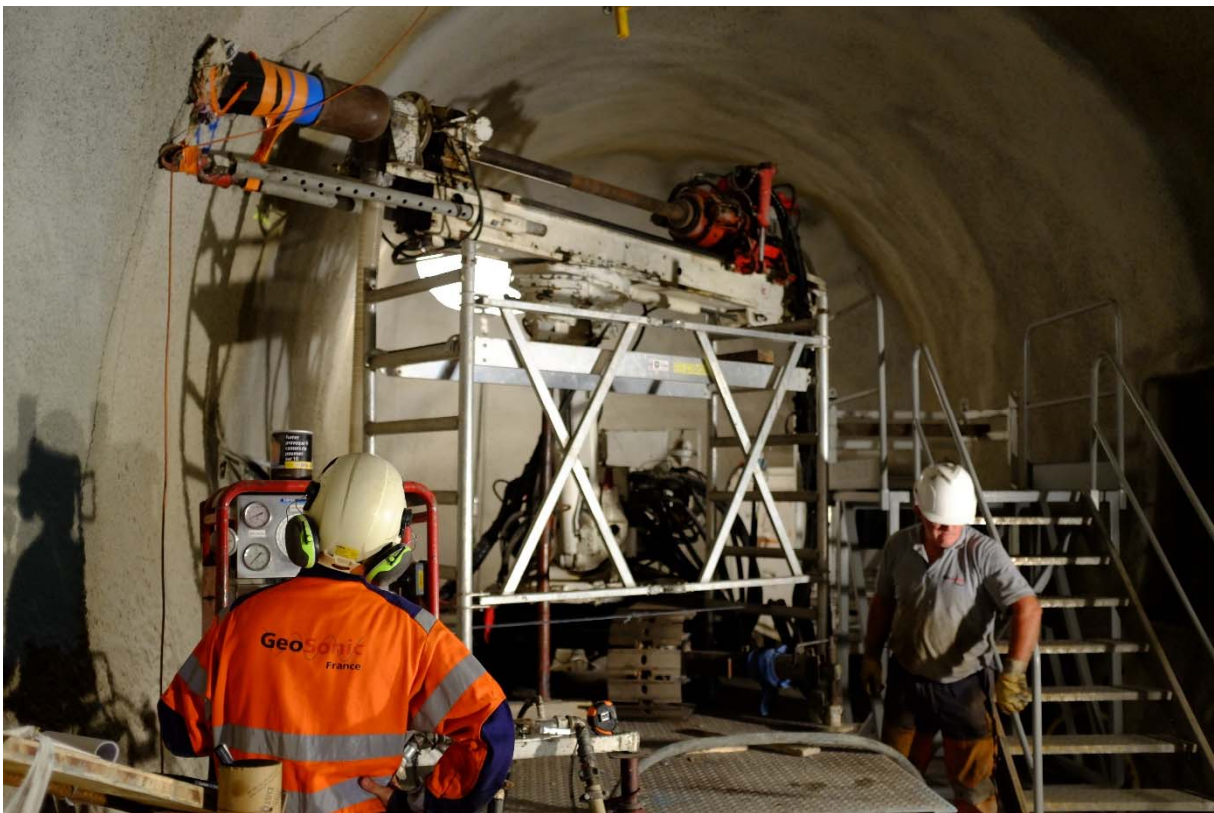
Figure 5: MB-A experiment: Geosonic drilling BMB-A9 with the help of a podium (Photo: R. Raselli, swisstopo).
