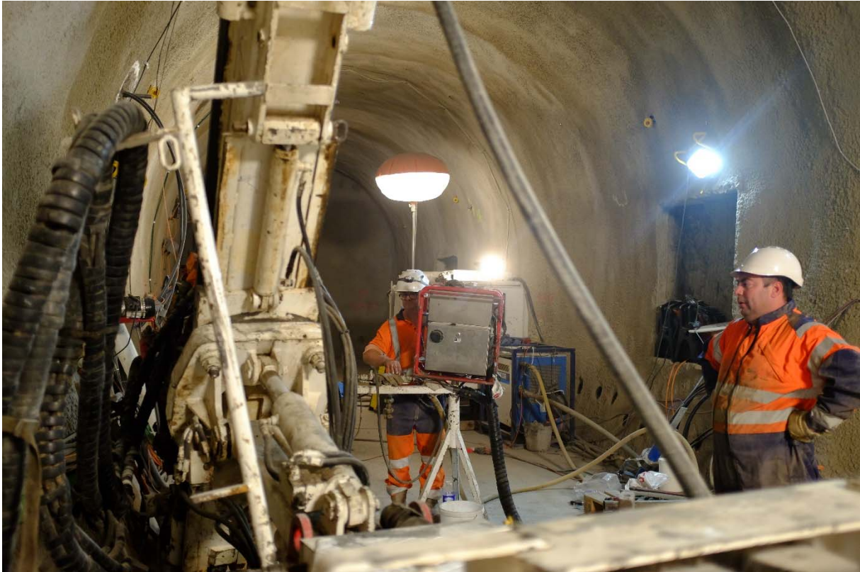
Figure 1: CS-D: The team of GeoSonic drilling borehole BCS-D5 (Photo: S. Schefer, swisstopo)
