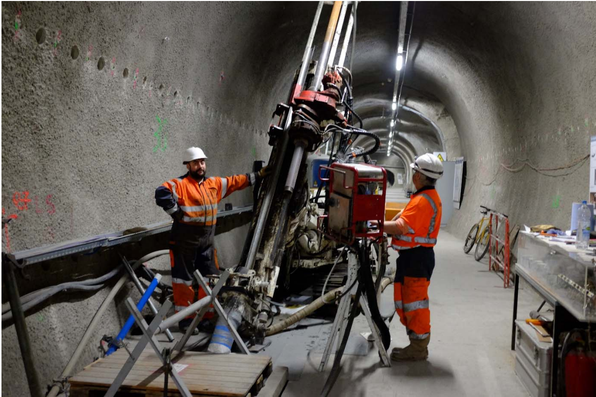
Figure 3: FS-B: J. Dubois and E. Parsy (GeoSonic) drilling borehole BFS-B4 with wireline technique (Photo: S. Schefer, swisstopo).
