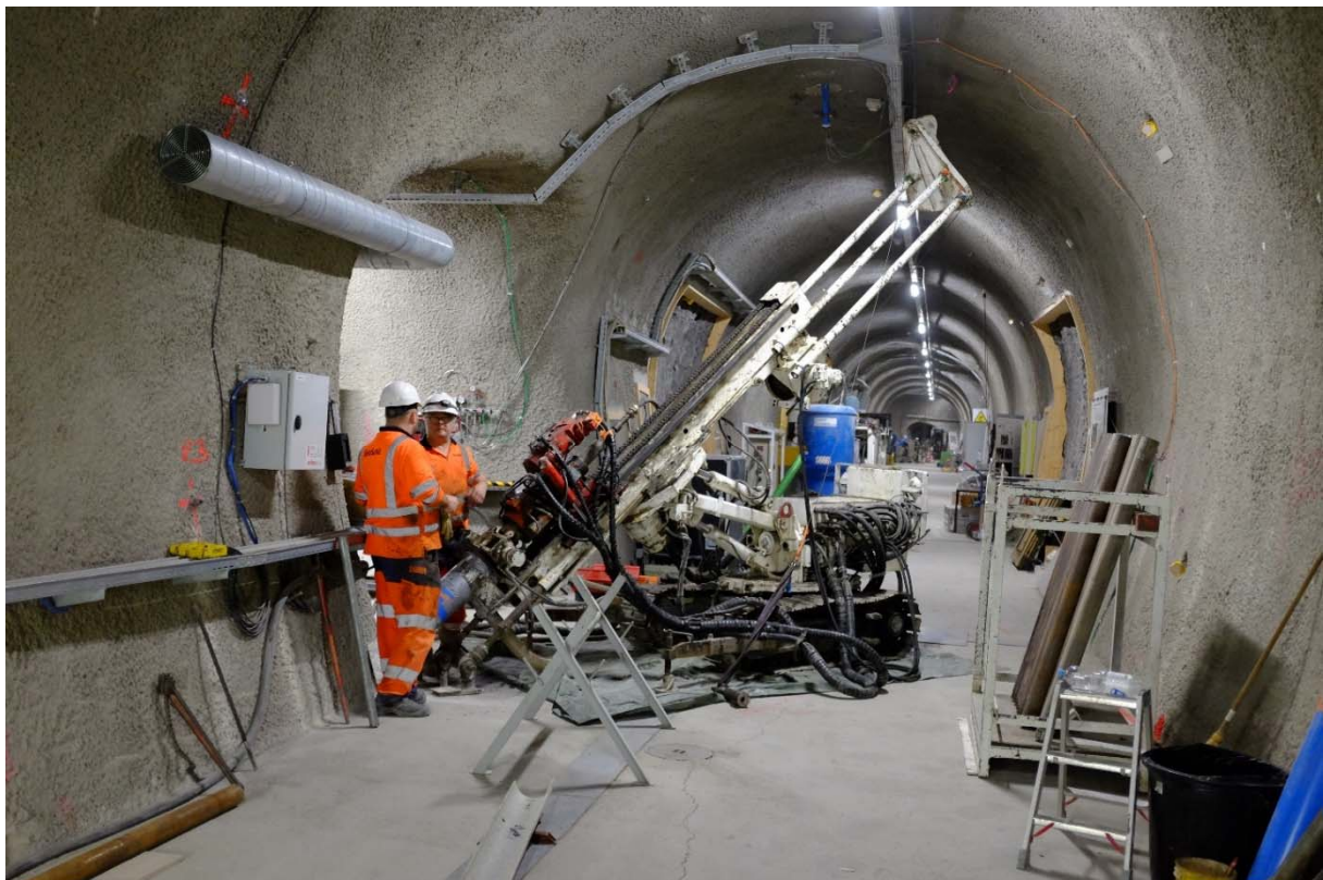
Figure 4: FS-B: GeoSonic drilling the first 25 meters of borehole BFS-B5 in Gallery08 (Photo: R. Raselli, swisstopo).
