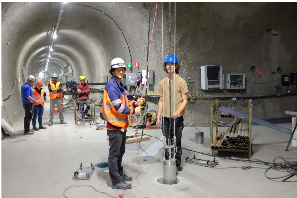
Figure 1: DR-B: N. Dietler (swisstopo) and M. Jaquenoud (Nagra) lowering an XRF-probe into the borehole BDR-B6 (Photo: R. Raselli, swisstopo).
