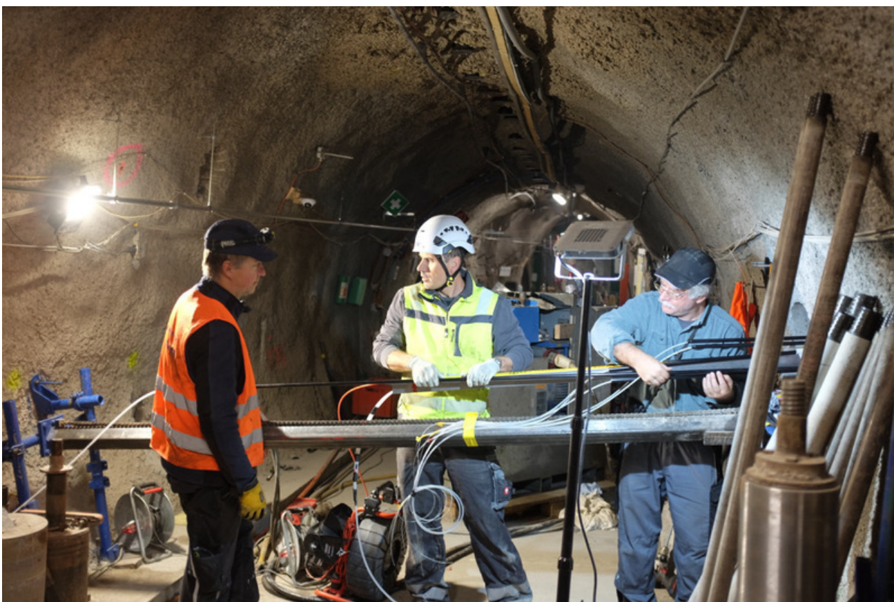
Figure 2: HE-E: The drilling support team inserting the needles for the resin injection (S. Schefer, swisstopo).
