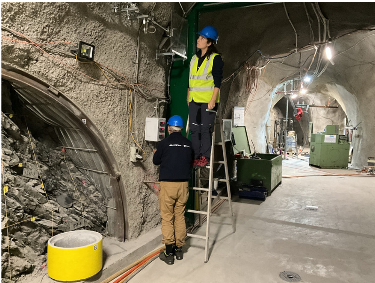
Figure 4: SM-C: I. Gutierrez and E. Meier (EMP) preparing the calibration of the hydrostatic-leveling system (HLS) (J. Windisch, swisstopo).
