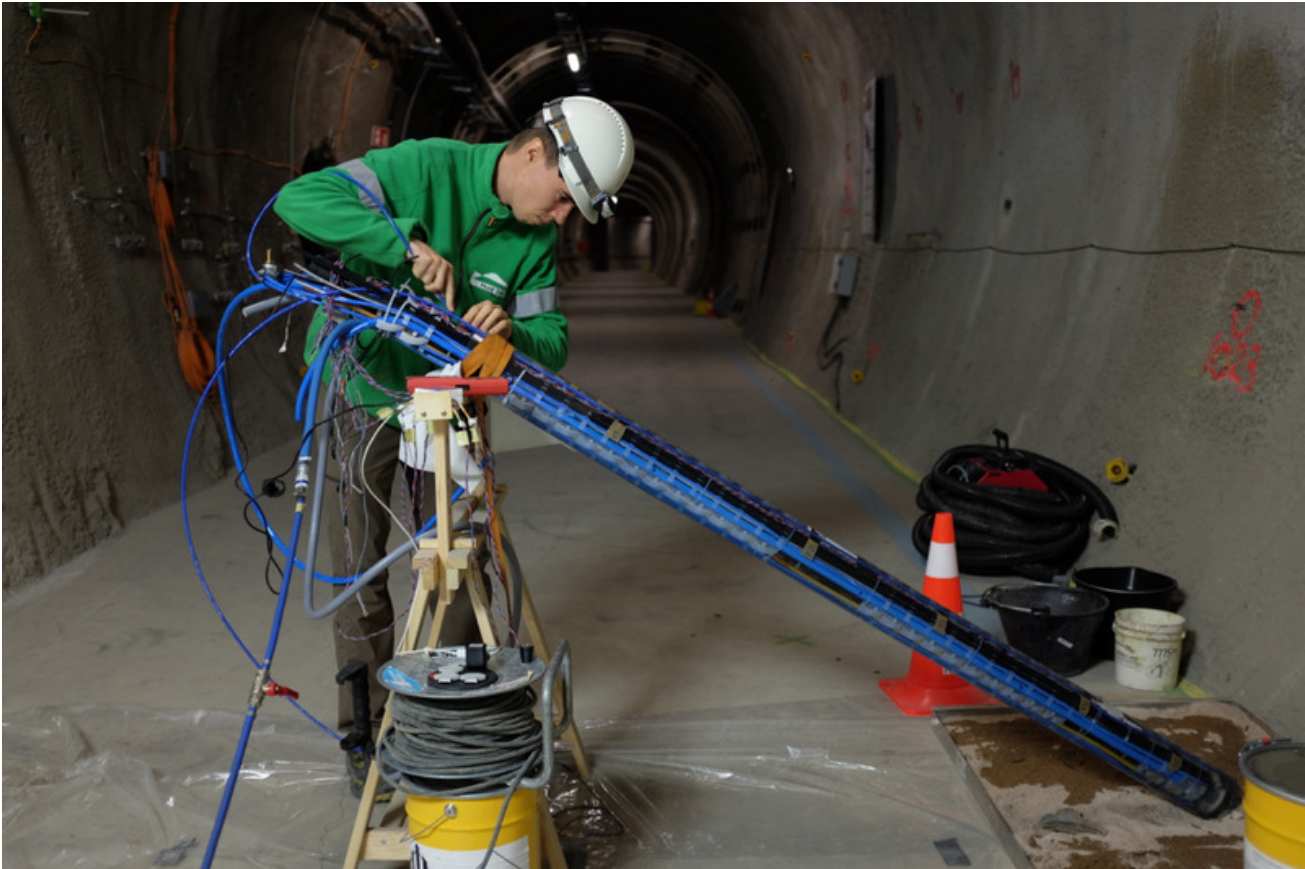
Figure 2: CL: J. Windisch (swisstopo) checking if the resin is cured (A. Grignaschi, swisstopo).
