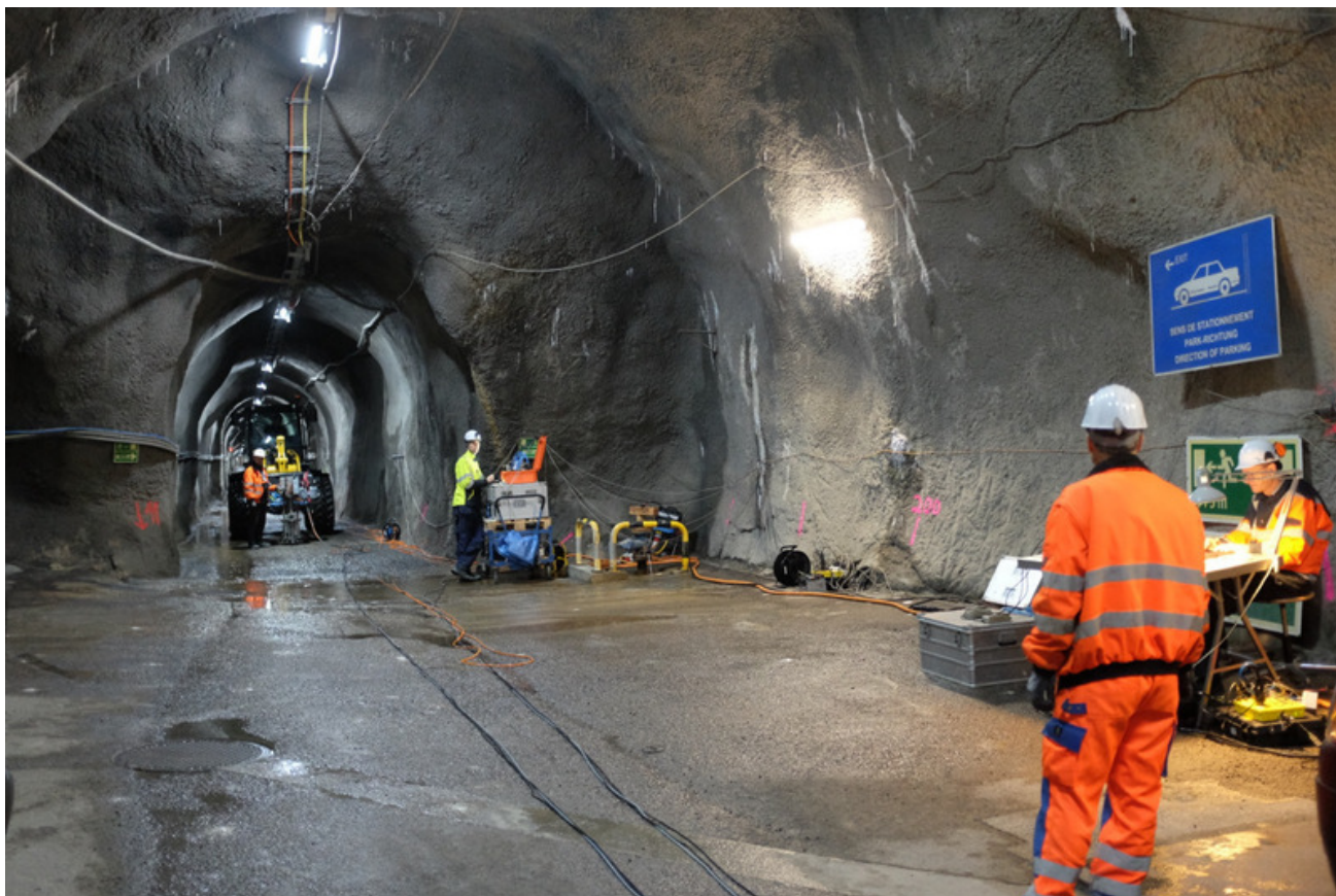
Figure 4: SI-B: Seismic measurements in the Safety Gallery (J. Windisch, swisstopo).
