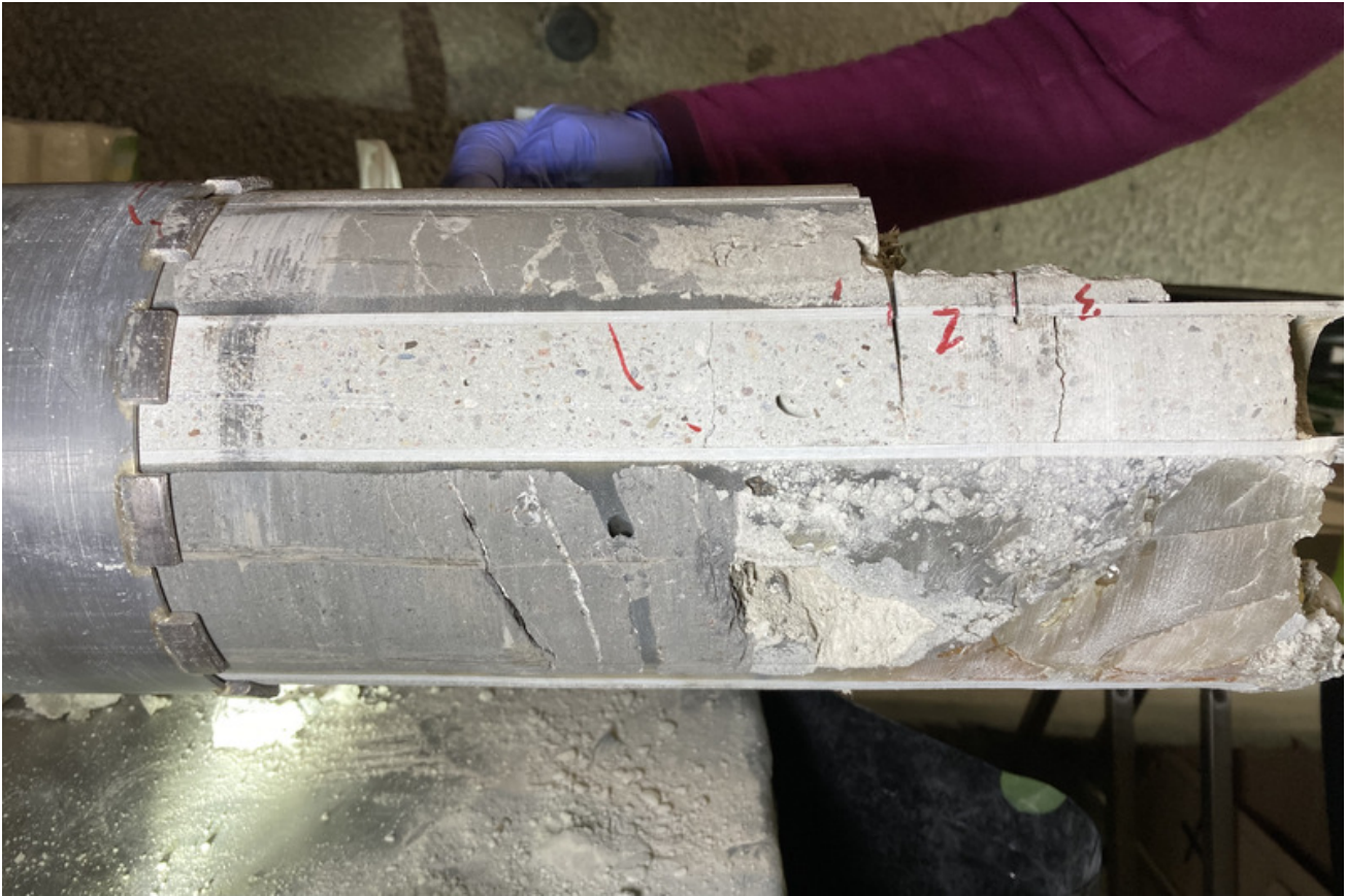
Figure 3: HE-E: Beautiful core from the interface between Opalinus Clay and bentonite close to the heater. The stabilizing drillings filled with resin are also visible (S. Schefer, swisstopo).
