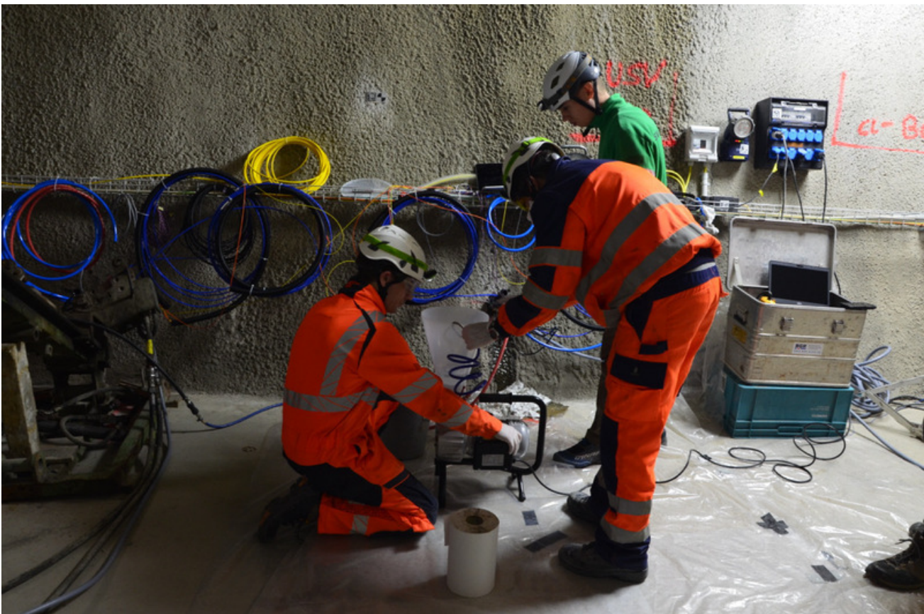
Figure 5: CL: Resin injection in BCL-4 (A. Grignaschi, swisstopo).
