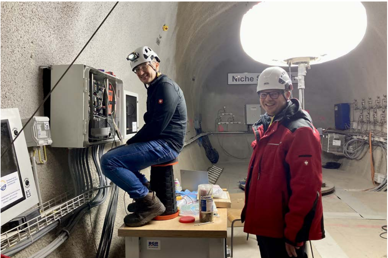
Figure 4: SW-A: Replacement and testing of the palatines for the ERT measurements (S. Schefer, swisstopo).
