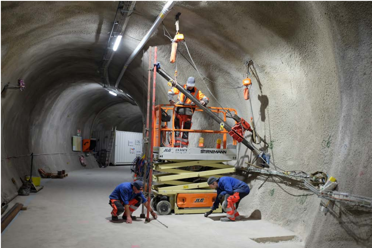
Figure 1: CL: Installation and orientation of the drilling rig (S. Schefer, swisstopo).
