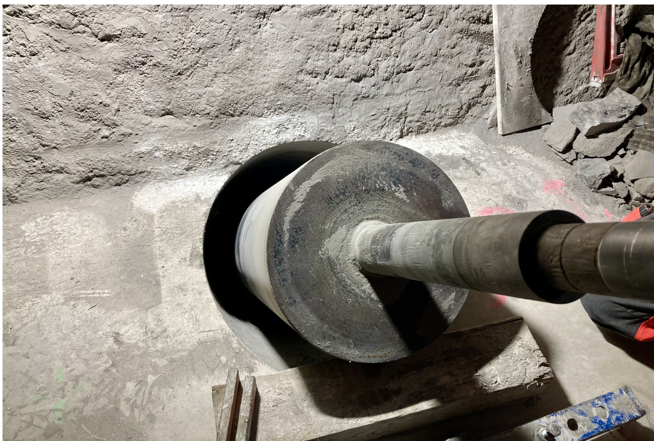
Figure 2: DR-D: The core barrel (400 mm) for the first 4 m of BDR-D3 (S. Schefer, swisstopo).
