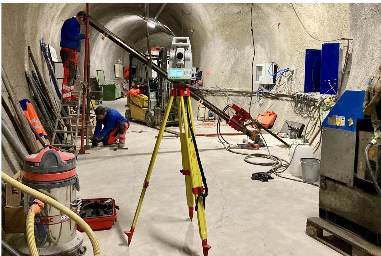
Figure 2: CL: The drill rig is perfectly parallel to BCL-5 (S. Schefer, swisstopo).
