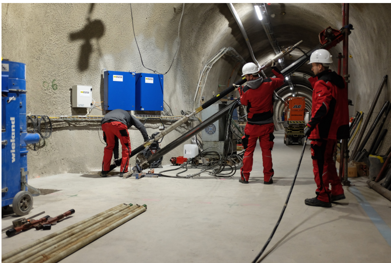
Figure 4: CL: Inserting the heavy pneumatic probe into BCL-7 is a team effort (S. Schefer, swisstopo).
