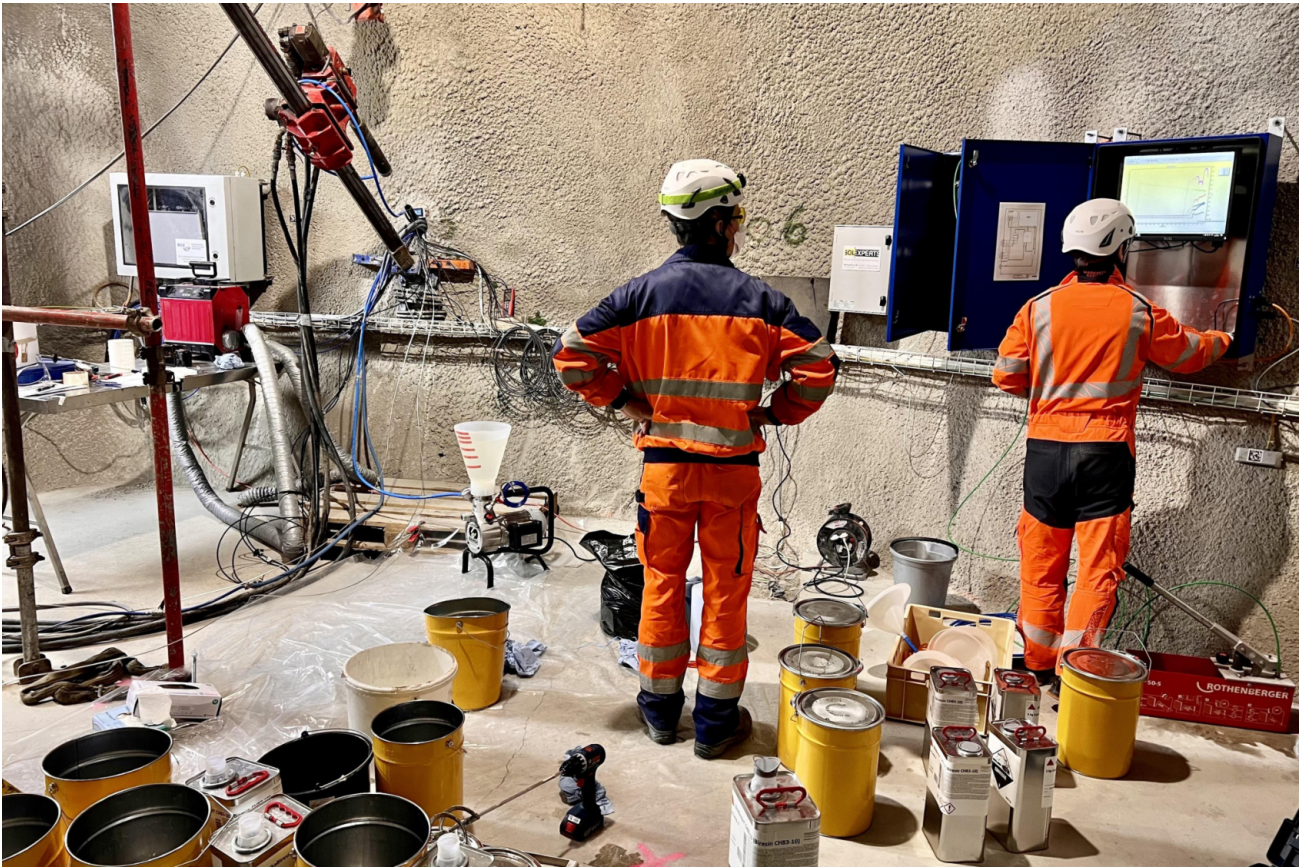
Figure 6: CL: Resin injection for BCL-5 (J. Windisch, swisstopo).
