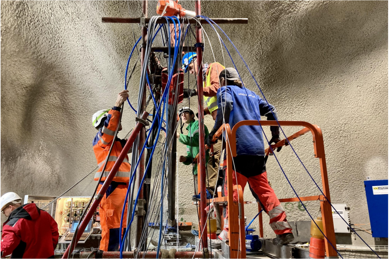
Figure 5: CL: Installation of the MMMS inside BCL-5 (S. Schefer, swisstopo).
