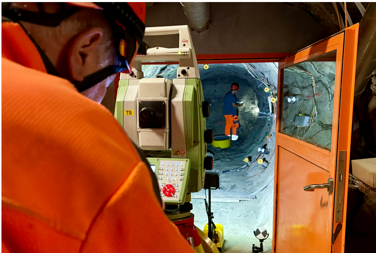
Figure 1: CD-A: Laser scanning inside the Closed Niche (S. Schefer, swisstopo)
