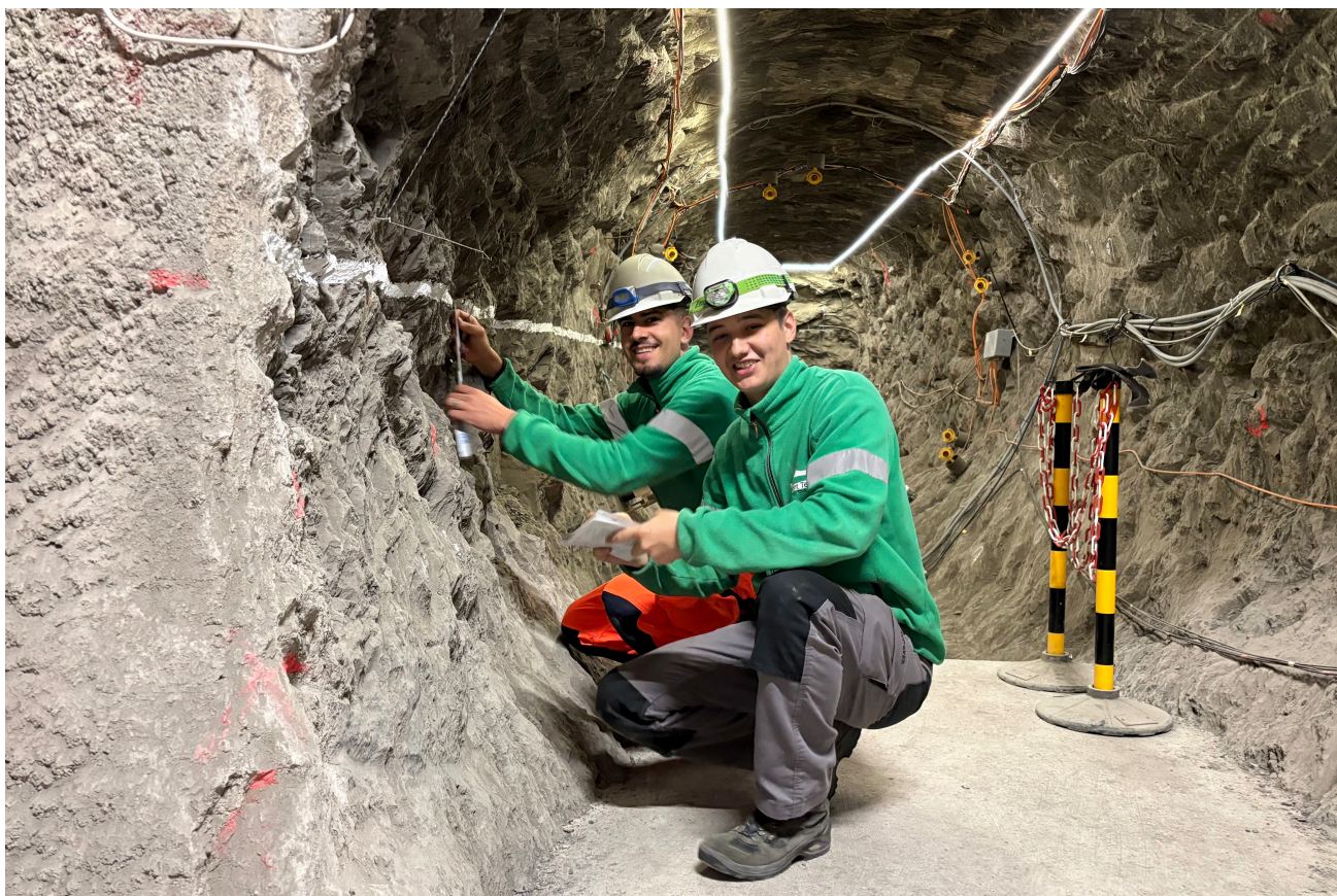
Figure 1: CD-A: Crack measures inside Niche Open Twin (S. Schefer, swisstopo)
