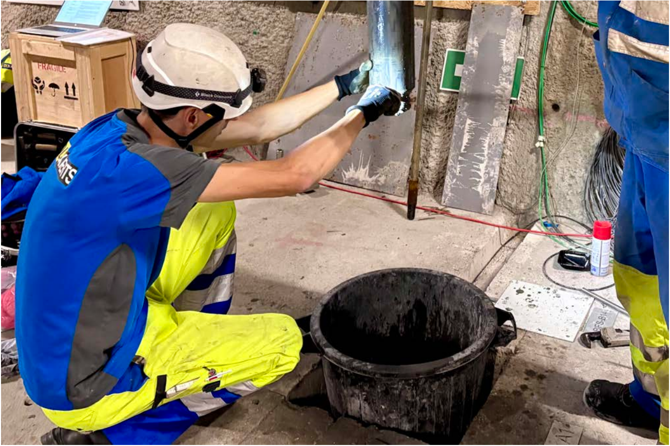
Figure 1: IC-A: Removal of the mud from the special screw tool by Solexperts. (J. Windisch, swisstopo)
