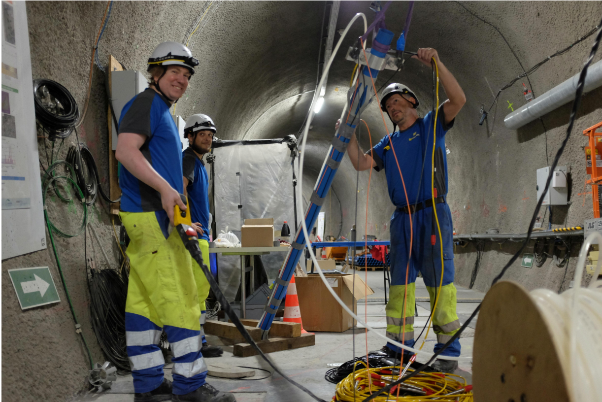
Figure 1: FS-B: The Solexperts team is installing the fibers behind casing (S. Schefer, swisstopo).
