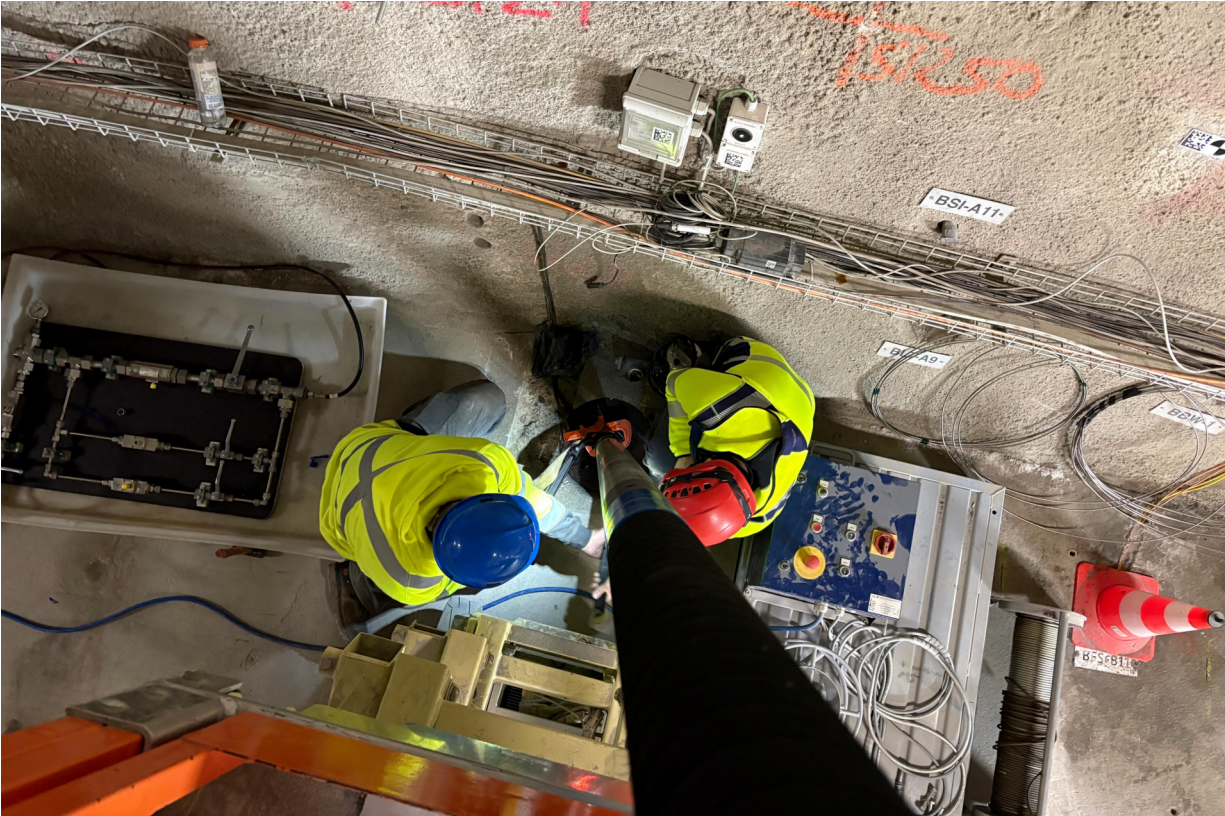
Figure 1: FS-B: Assembly of the packer system (S. Schefer, swisstopo).
