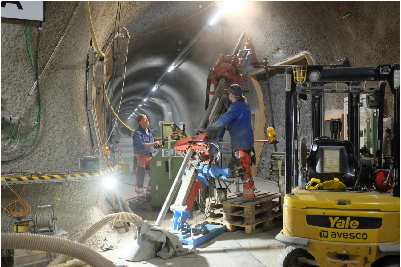
Figure 1: FS-B: At greater depth, getting the cores out becomes a real task (S. Schefer, swisstopo).
