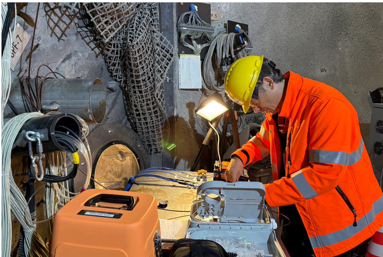
Figure 3: PF-A: Connection of the fibers from BPF-7 to the connecting cable for Niche CO 2 (S. Schefer, swisstopo).
