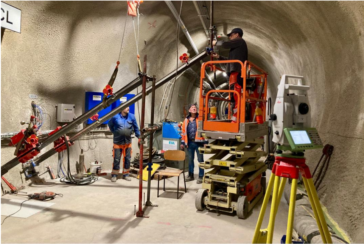
Figure 1: CL: Orientation of both rigs to be parallel within 0.1 degrees takes a lot of patience... (S. Schefer, swisstopo).
