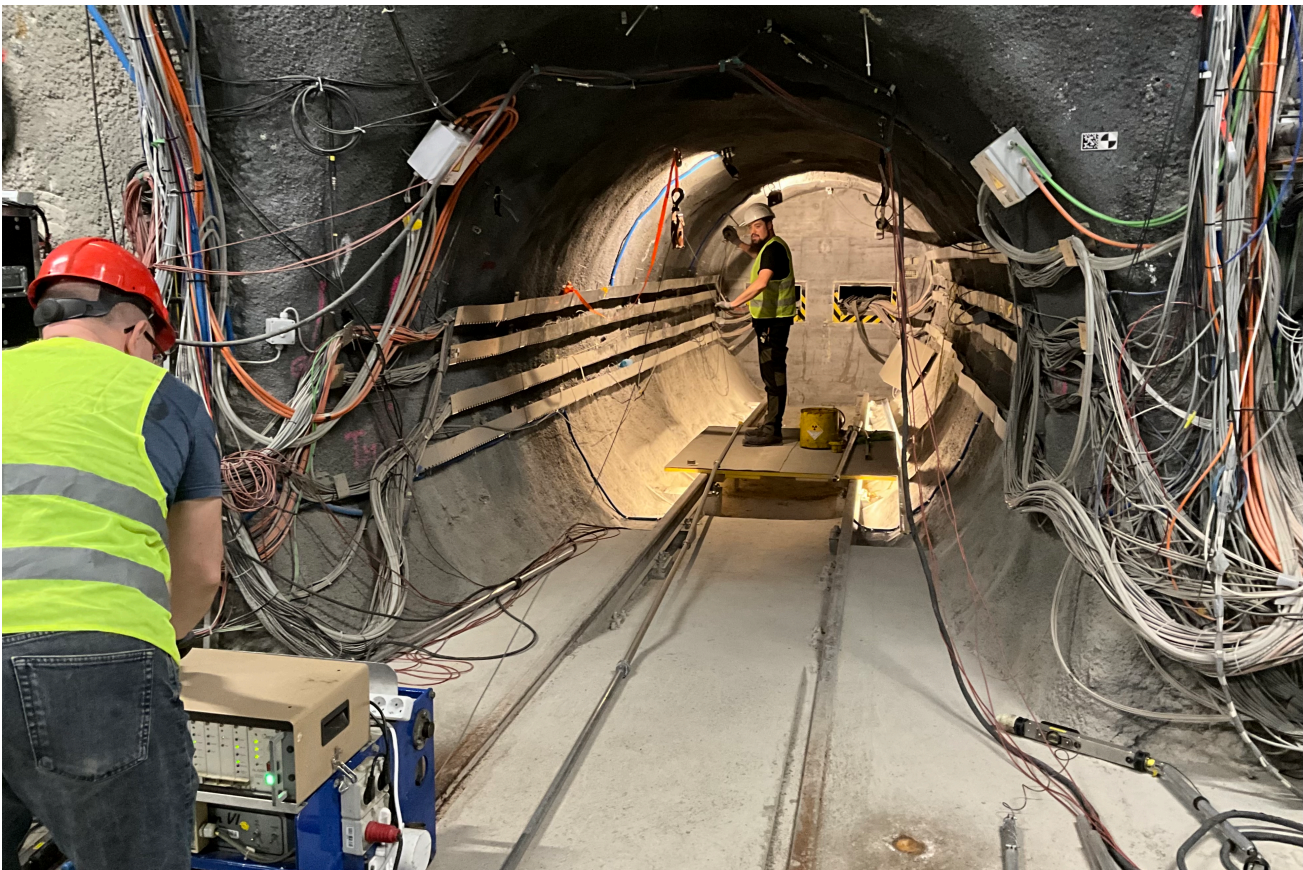
Figure 1: FE-M: Measuring density inside GT-1 (S. Schefer, swisstopo).
