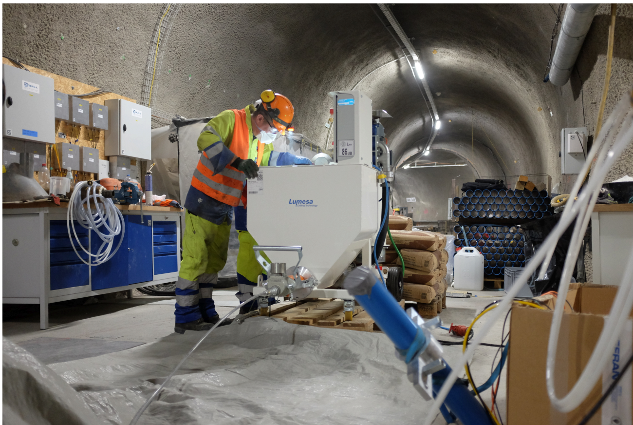
Figure 2: FS-B: Injection of the Pumice cement into BFS-B13 (S. Schefer, swisstopo).
