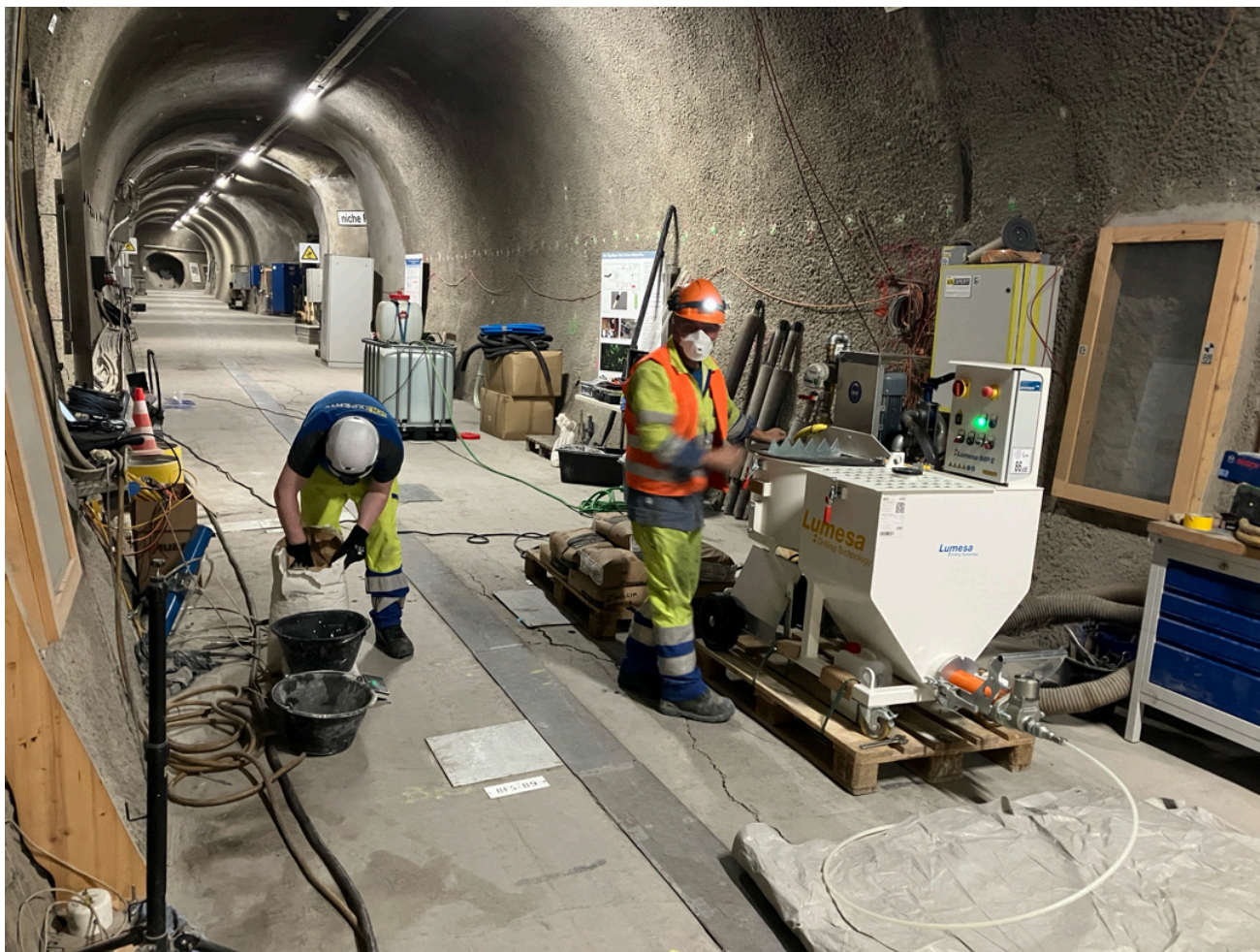
Figure 2: FS-B: Solexperts team performing the grouting (S. Schefer, swisstopo).
