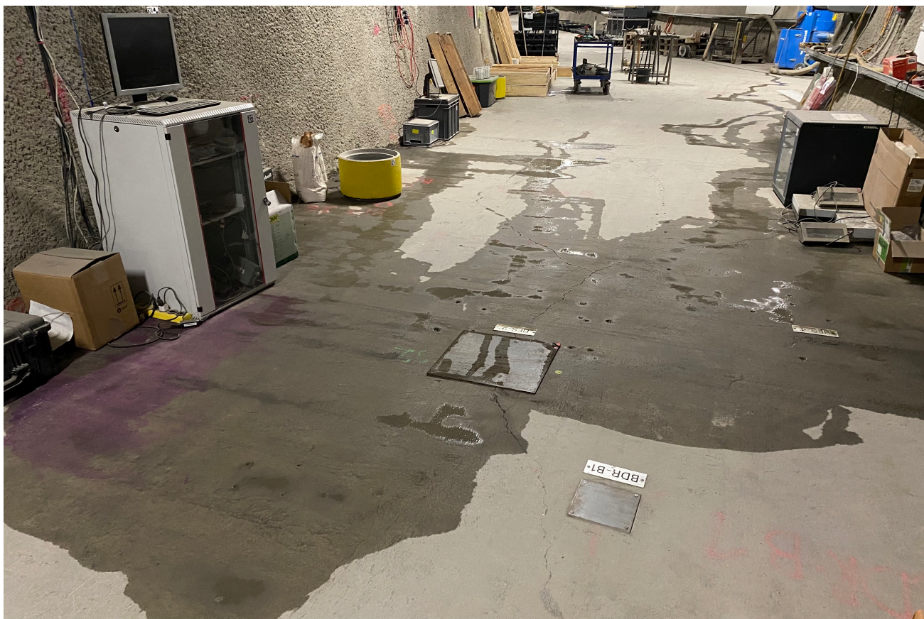
Figure 1: FS-B: Water pushed out from the existing boreholes (M. Ziegler, swisstopo).
