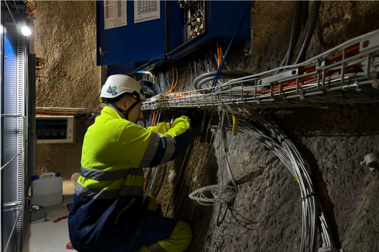
Figure 1: CL: Fixing the new flow lines for the injection (S. Schefer, swisstopo).
