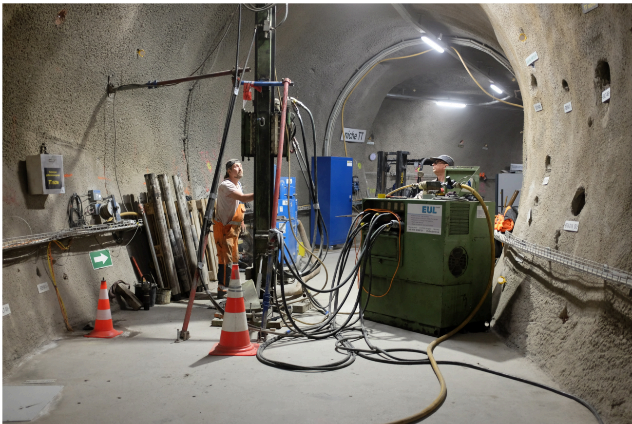
Figure 4: FS-B: Drill rig for BFS-B15, vertical borehole (M. Abdelouhabi, swisstopo).
