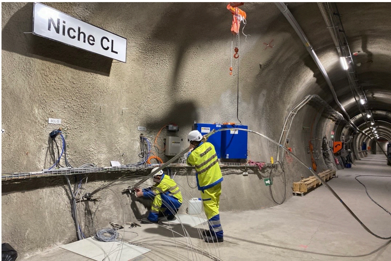
Figure 3: CL: Installation of the hydraulic multi-packer system for geochemical sampling and pore pressure monitoring at BCL-10 (M. Ziegler, swisstopo).
